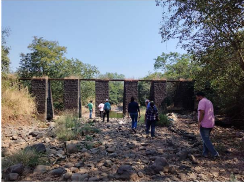
Picture 5.1: Non-functional KT weir on one of the main streams in the catchment:
