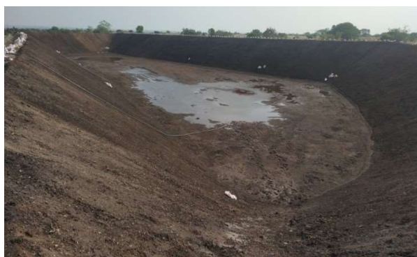
A huge farm pond under construction in Kumbhefal village
